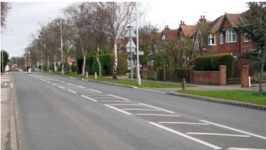
Soakaways set beneath the grass verges return surface water run-off from the carriageway to ground at a safe rate.
