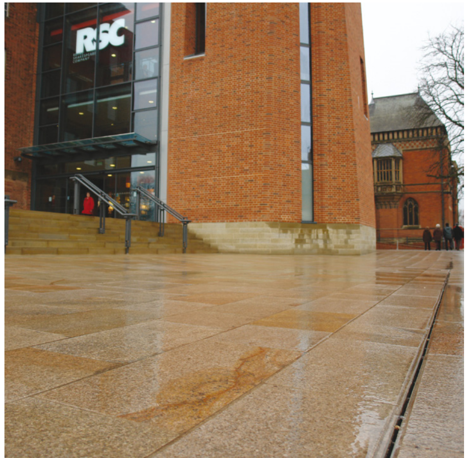
The 10mm Brickslot inlet allows apparently unbroken surfaces to be created.
