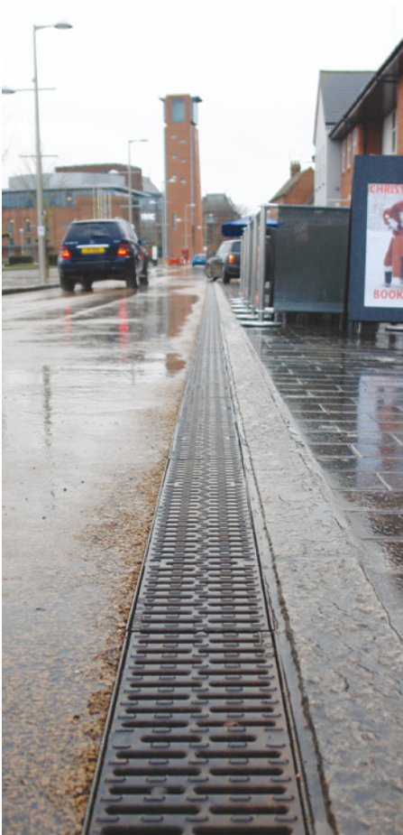
Cast iron gratings harmonise with the heritage street setting.
