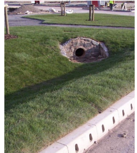
Maintaining a grass height of 50mm optimises primary filtration within the swale.
