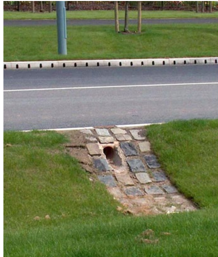
The shallow inlet created by using KerbDrain 305 has minimised swale depth.
