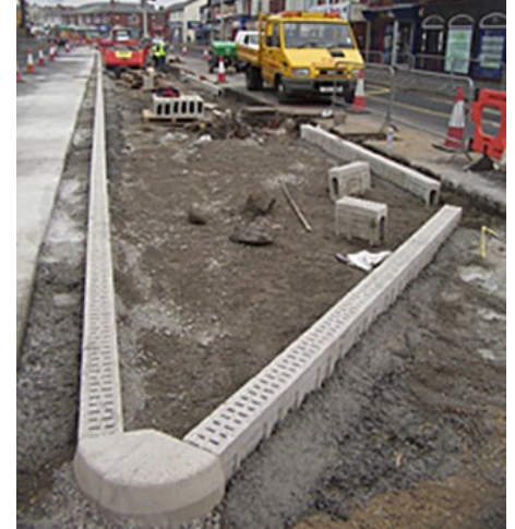
Installation of ACO Products.
