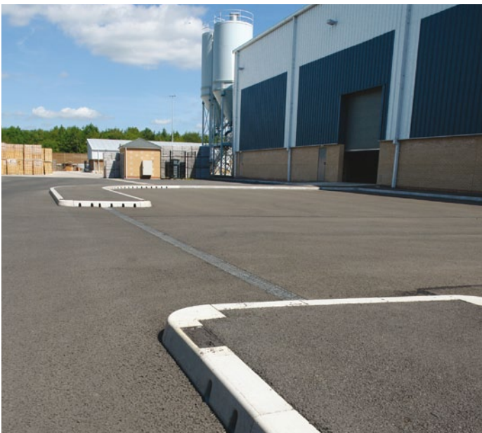
The staff car park is edged using the award winning ACO KerbDrain combined kerb drainage system.
