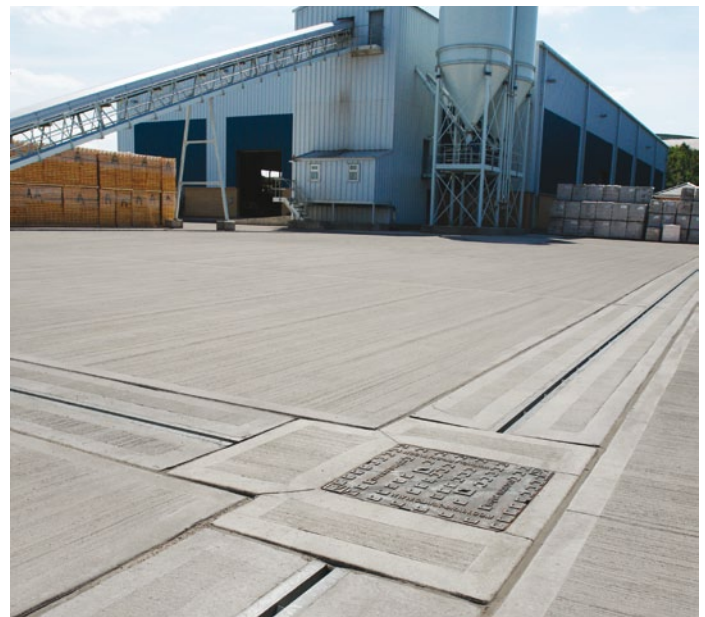
Heavy duty edge rails fitted to the ACO Qmax runs securely anchor the inlet to the surrounding pavement, helping give the system Load Class F900 performance.
