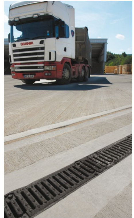
ACO’s heavy duty S-Range grated channel system has been installed in the highly trafficked vehicle wash-down area.
