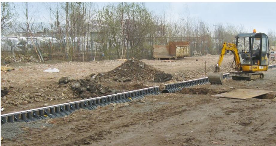
A single run of ACO Qmax has replaced the original point gully design, minimising ground infrastructure, installation time and costs.
