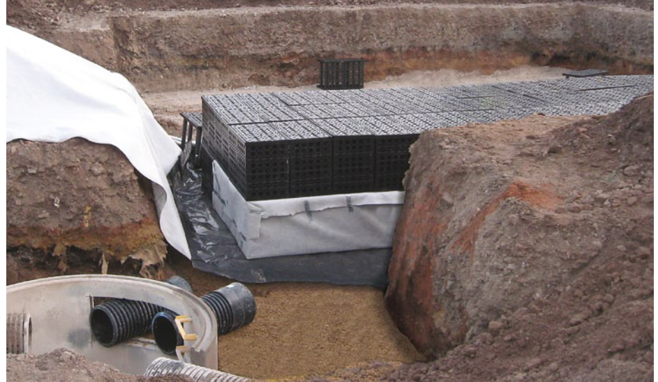
The combined attenuation provided by the ACO StormTank and ACO Qmax allows the site to operate under maximum storm conditions.
