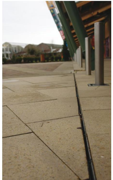
*To create the impression of an unbroken paved surface in visually sensitive pedestrian areas the architect has specified ACO Brickslot.*
