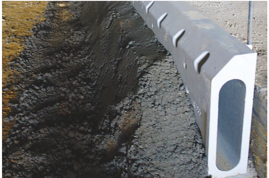
The 45 degree Splay profile on the ACO KerbDrain 480.
