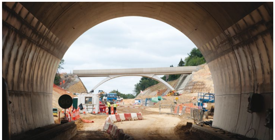
* Work commences on the Miss James footbridge.
