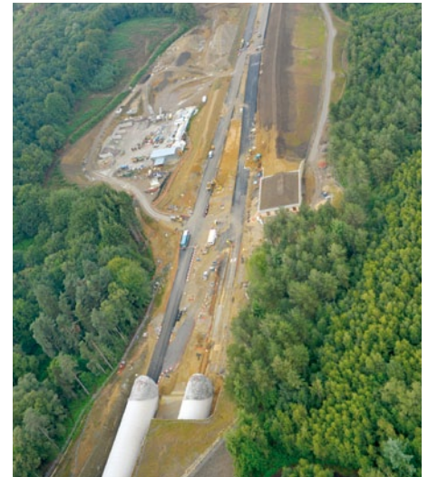
* The Hindhead tunnel from above.
