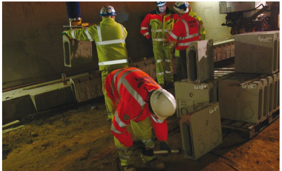
Ease of sealing and handling allow lay rates in excess of 300m a day.
