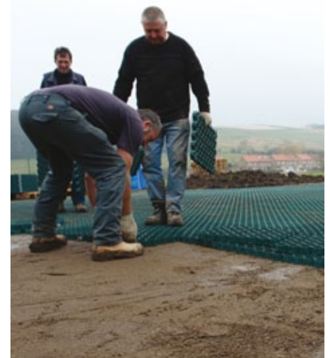
ACO GroundGuard installation.
