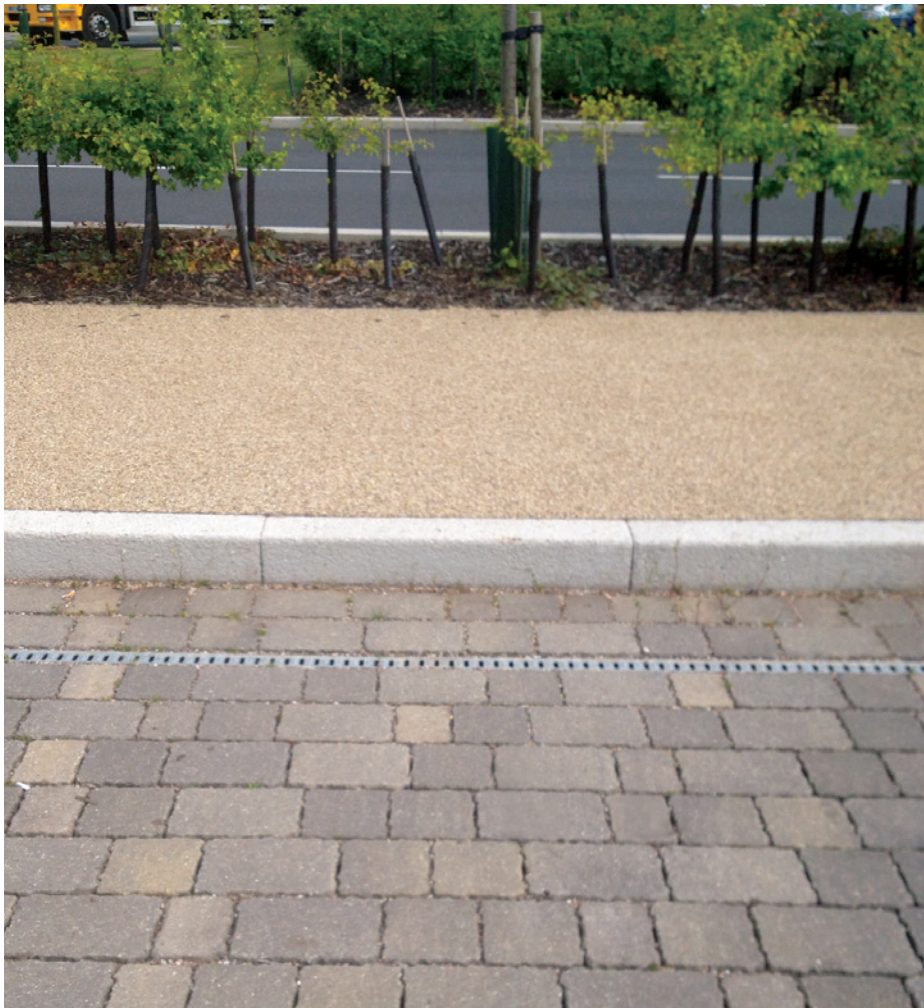
ACO Qmax® Slot drainage system manages exceedance during heavy downpours.
