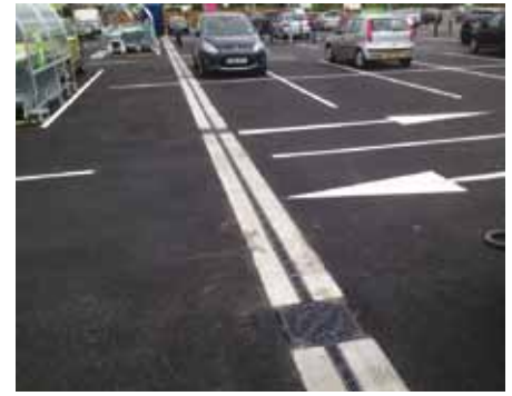
Surface water interception via 90m run of ACO Qmax
