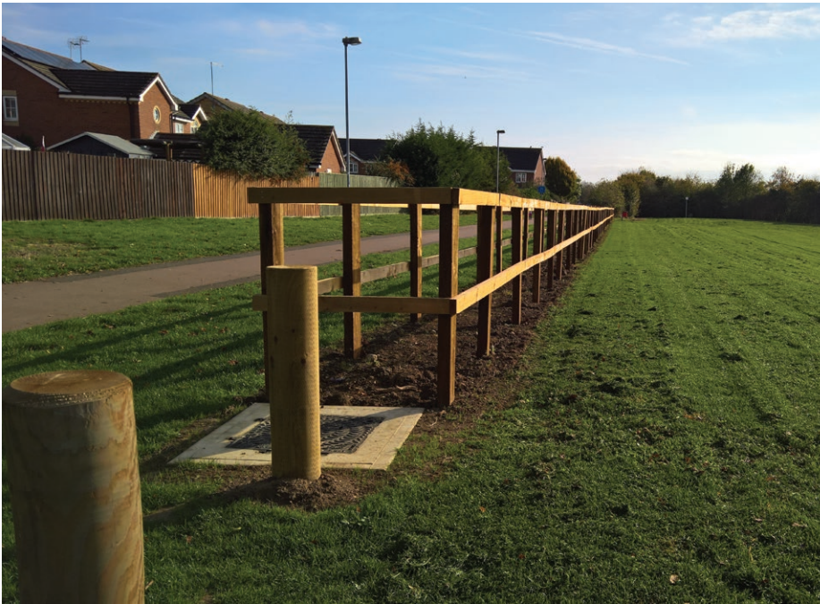
Narrow ACO StormBrixx configuration at the end of playing fields with man access cover
