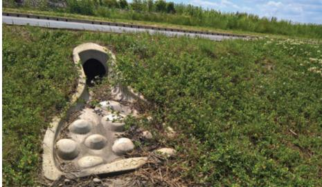
designed to link proprietary conveyance drainage systems, such as KerbDrain, to vegetated infiltration features. The ACO SuDS Swale Inlets had outfalls at 10m centres along the A12, to discharge the surface water via infiltration into the subsoils of the Swales.
