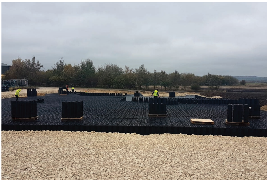
ACO StormBrixx SD being installed
