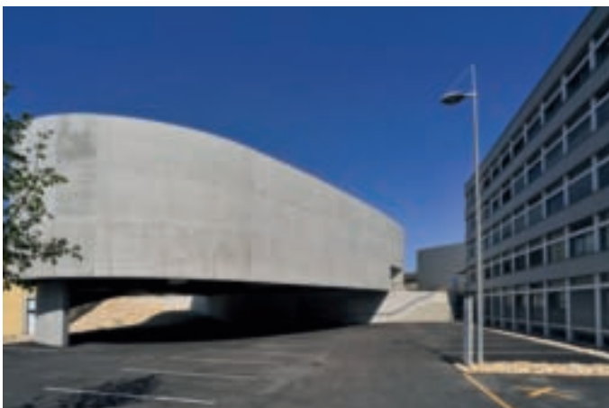
Laufen Company near Basel, Switzerland [2012]
