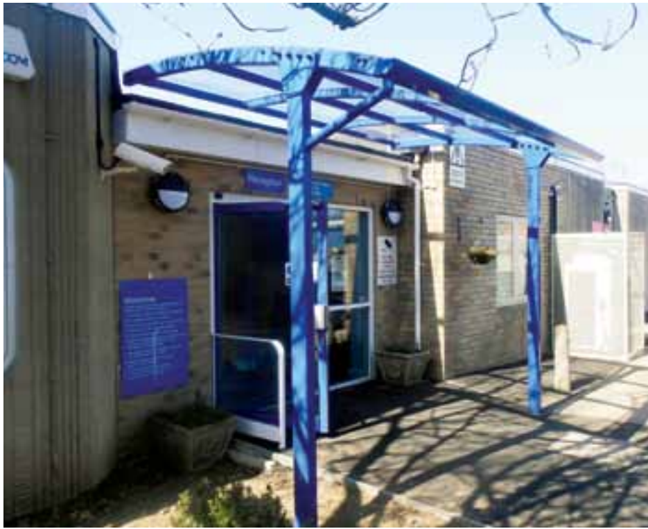
Steel legs supporting timber roof
