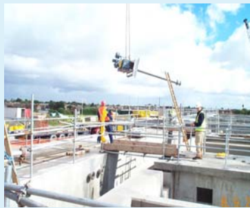
Actiflo Plant during construction
