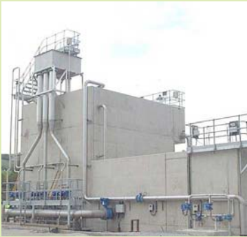
Biostyr Plant frontal pipework including dirty washwater storage tank
