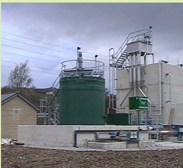
View of MCC room and Kalic storage and dosing plant
