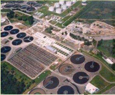
Aerial view of Biostyr Plant located between ASP1 lane and storm drain culvert
