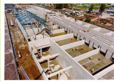
Biostyr Plant during construction
