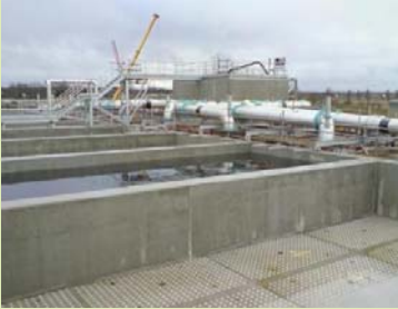
Biostyr Cell Filter Floor (during construction)
