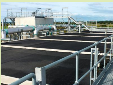
Biostyr plant – Plan View above Filter Cells
