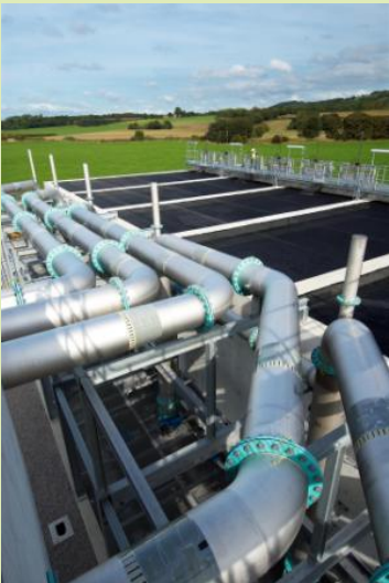
Biostyr Raw Water Feed Pipework
