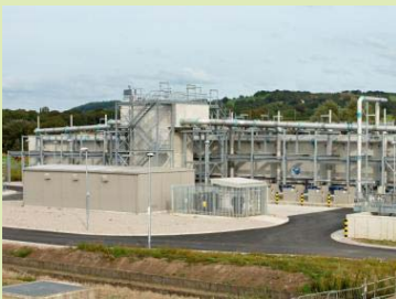
Biostyr Plant – Front Elevation
