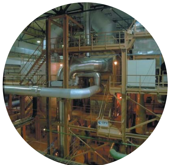
Saint-Petersburg (Russia) - The PYROFLUID™ incinerator combined with thermal exchanger
