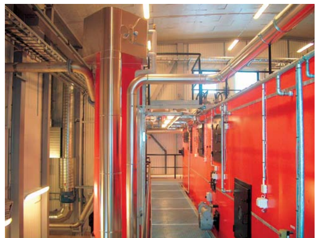
BIOCON™ energy recovery plant at Mora (Sweden)
