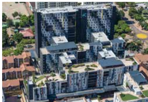
Hatfield Student Apartments, Pretoria, South Africa
