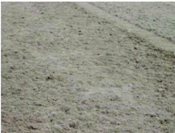
Levelling reinforced Fibresand
