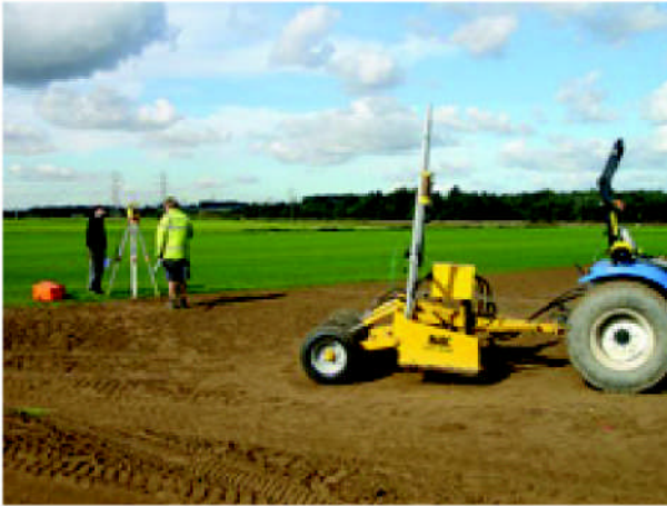
Laser levelling of surface
