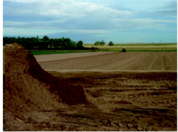
Laying of reinforced fibresand
