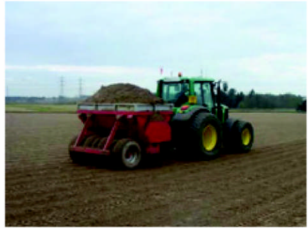
Laying fibre reinforced sand
