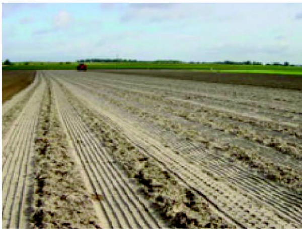
Laying reinforced Fibresand
