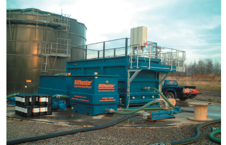
D100 DAF unit on food processing plant
