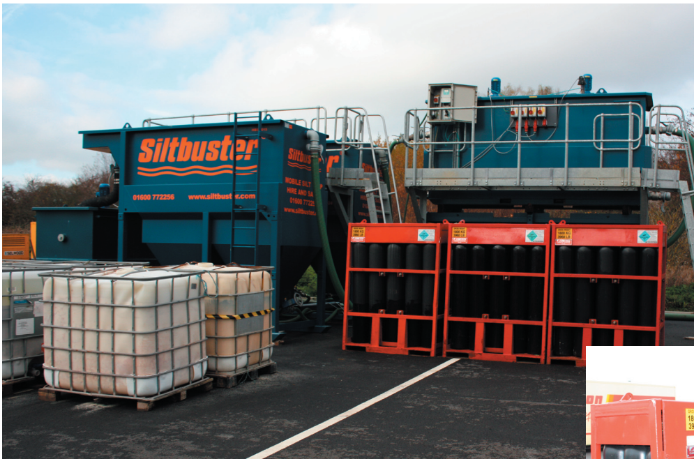
Three Stage pH Adjustment using Siltbuster treatment plant
