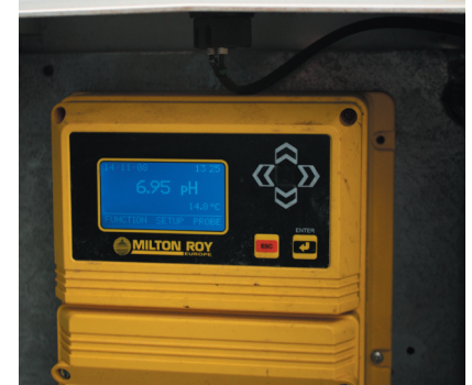
Automatic Adjustment and control of pH
