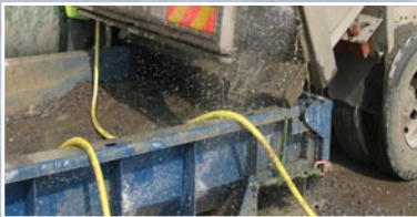
Low Level Trays (concrete pumps)
