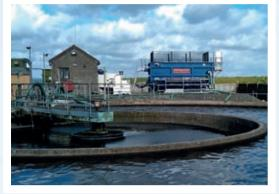
Whilst the use of DAF for sludge thickening applications is well documented, they are still relatively unused on municipal sites. DAFs are ideal for this type of temporary application because they are small and portable - they can be brought onto site and installed via lorry-mounted crane.
