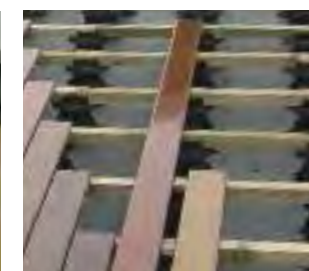
DPH5 pedestals used with joist cradles for timber decking
