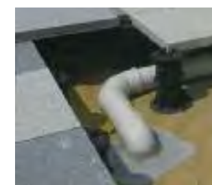
At roof level, DPH pedestals are used to support stone pavers to contain and protect the services for ventilation, water supply, lighting etc.
