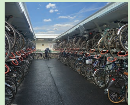
140 Josta 2-Tier Racks under the Cycle-Works Kennet Shelter
