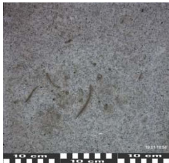
Typical Pavement Grime on a Granite surface
