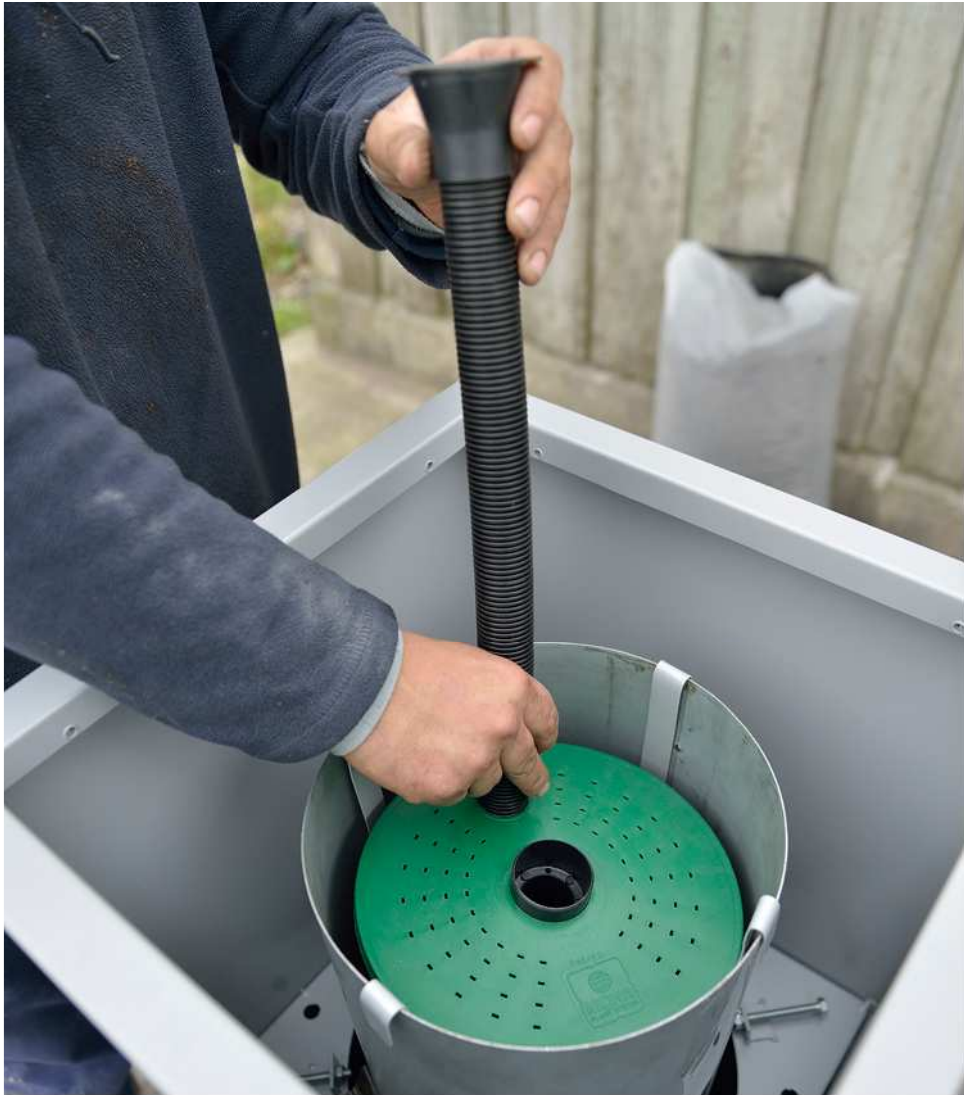
Step 8: Install the self-watering reservoir, placing it into its cradle within the bollard.
