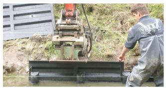
Push or drive the Technic panels behind the poles into the ground until the top of the Technic panel hits the top of the pole. Connect the Technic panels to the Combi-poles using torx stainless steel screws of 5 cm.
