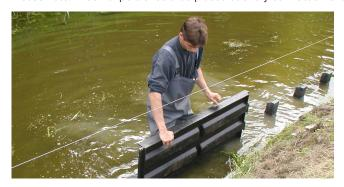
Install the Technic panels behind the Combi-poles and connect the Technic panels by sliding the panels into each other using the tongue and groove joint. The Technic panel is 1.40 wide. The Technic Curve panel is 0.5 meter wide and used for curves.
