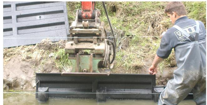
Push or drive the Technic panels behind the poles into the ground until the top of the Technic panel hits the top of the pole. Connect the Technic panels to the Combi-poles using torx stainless steel screws of 5 cm.
