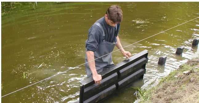
Install the Technic panels behind the Combi-poles and connect the Technic panels by sliding the panels into each other using the tongue and groove joint. The Technic panel is 1.40 wide. The Technic Curve panel is 0.5 meter wide and used for curves.
