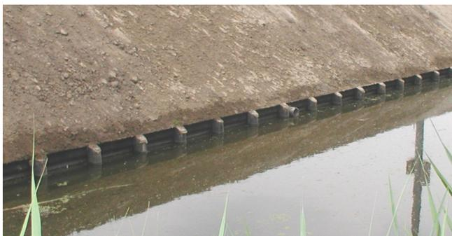
Back-fill with soil and level behind the Technic panels for a neat, sustainable finish.
