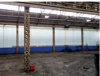
For the orignal installation, Westgate suggested their Flexiwall FR610 solution; manufactured in fire rated PVC materials and then suspended and tensioned using the existing buildings structure to form a permanent partition.
