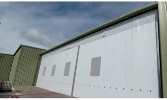
Westgate were approached by Don & Low Ltd to supply walling that could create a dust and weather tight seal on either side of a drive through area, which was between two production buildings at their site in Forfar, Scotland.
