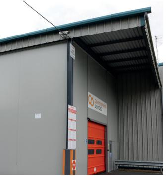
Westgate provided and installed a 10m x 10m external Flexiwall which was hung from the existing canopy roof structure. A Fastflex fast action door and a steel pedestrian door were also supplied and installed by Westgate.
