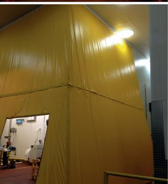
In this most recent project, Birds Eye were tasked with carrying out some works to an existing process area at their factory in Lowestoft. This involved removing some existing masonry walls and installing new walls and doors. All of this needed to be achieved without contaminating the existing process plant.
