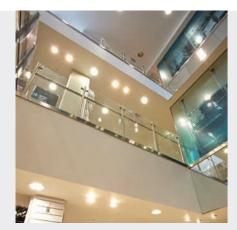
specified Onyx balustrades to the customer staircase, escalator void and gates leading to window display areas. The installation is notable ISG Retail & Leisure for the D-shaped lugs used in place of 'banjos'.
