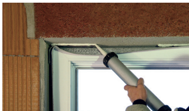
Installation example: ISO-TOP FLEX-ADHESIVE SP
