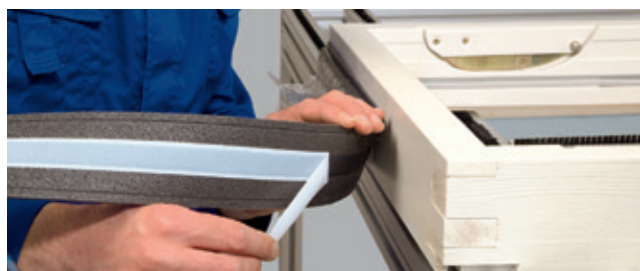
Installation example (1-BT): Fitting wooden windows
