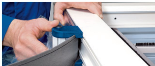
Installation example (CB): Fitting PVC windows
