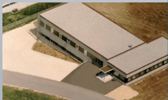
The company’s first purpose-built production and administration building is opened in Röntgenstraße in Aalen.
