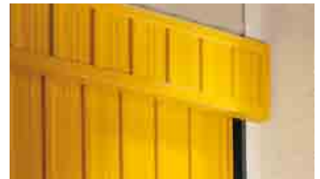
Detail of upper transom of Mono sectional door (flush-mounted).
