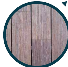
Weathered, cleaned decking
