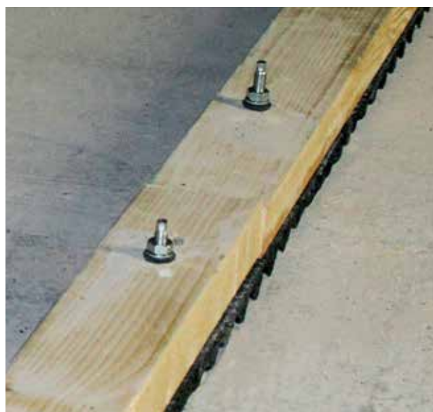
Elastic washers with and without centring aid (groove)
