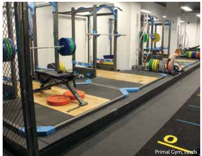
Constructing a floating floor for Primal Gym, Leeds
