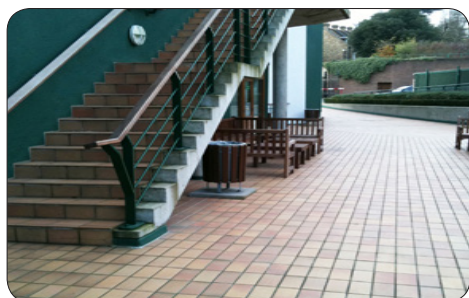
Before: the terrace flexed due to heat expansion and contraction, causing the tiles to lift.
