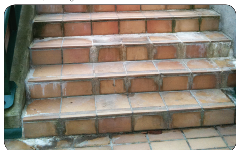
Before: cracked, frost damaged and stained tiles
