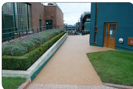
After: smooth, safe permeable resin-bound paving
