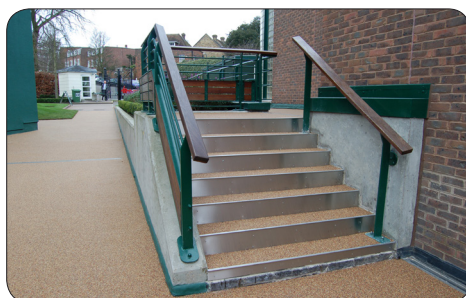
After: steps with stainless steel risers, in-filled with resin-bound paving, which will not tarnish or corrode over time
