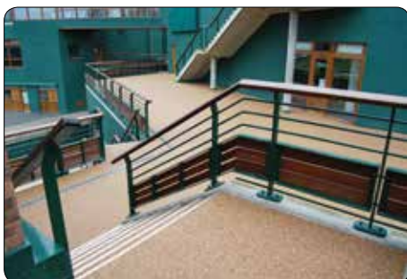
Wimbledon AELTA: Press area private roof terrace and steps. Wimbledon, London
