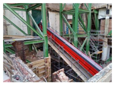
The demolition of the entire building whilst retaining the facade created a challenge when removing all the demolition rubble through the listed facade from the existing basement and into the back of a muck away truck which was parked in a closed road to the side of the building. Also, with a limited program for works, the rubble had to be removed as fast as possible.
