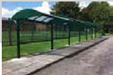
Sacred Heart School, Newry Covered Walkway
