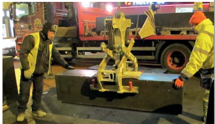
Offloading and installation of Blyth bench using grab-lift
